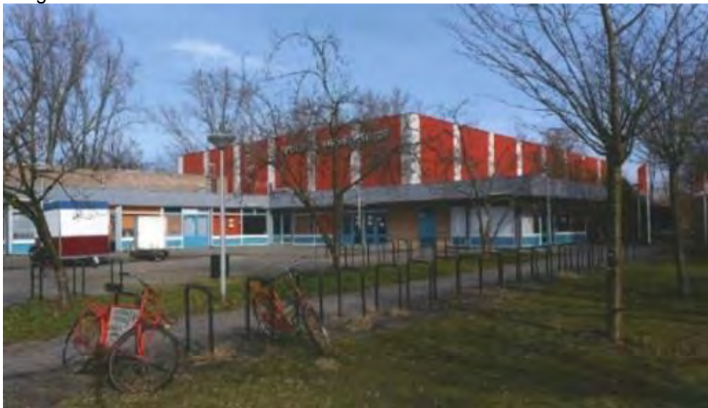
Entree: asfalt, auto's, hek
